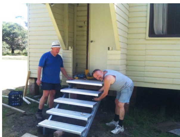
Installing new steps at Vijayaloka: Tim Lamble and Kevin Griffith
